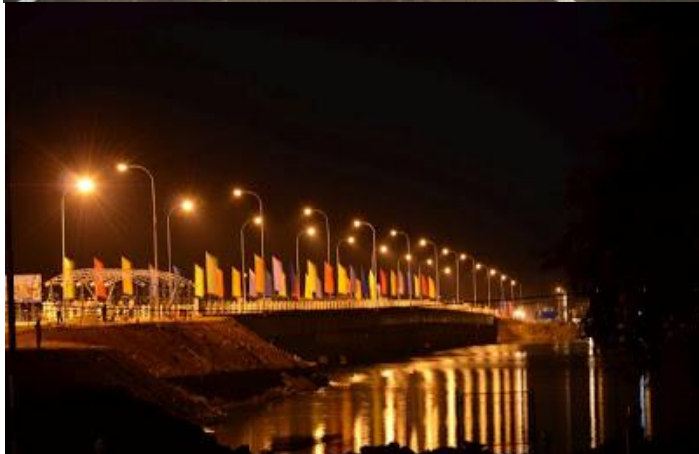
The New Bridge by day and by night courtesy: battinews.com
